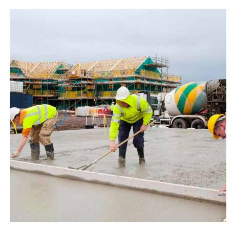
Used in conjunction with a standard open panel timber frame system at Saxon Park, Insulslab offered improved airtightness as the two systems integrated well to virtually eradicate thermal bridging at the junctions.
