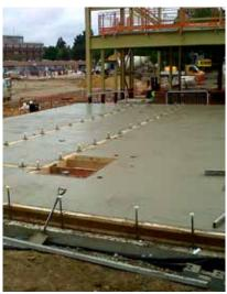
With speed of build a key consideration in the custody suite programme, Insulslab was used in combination with precast concrete walls. As a flexible specification, the Insulslab profile was designed with recessed channels, allowing the precast walls to be easily positioned in place.
